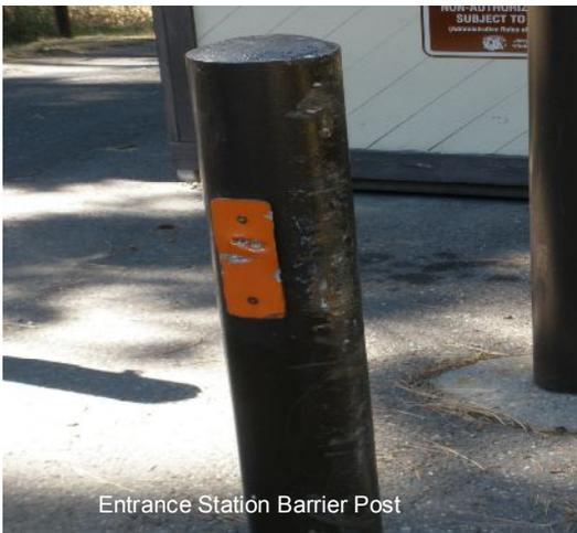
The present entrance to the park was designed for smaller, shorter vehicles, and hence the turning radius is now insufficient for the more common larger RVs in the 32-36' length range. The current entrance turning radius is too tight, and many towed vehicles have left their mark on the barrier posts that protect the entrance station.
