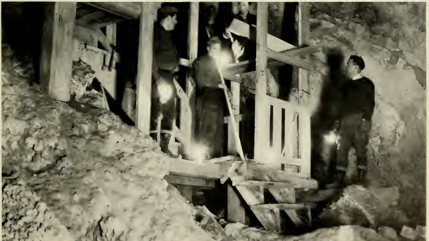
The Civilian Conservation Corps installed new stairways and an electrical lighting system in Lewis and Clark Caverns during the 1930s as part of a $2 million improvement. photo: courtesy National Park Service
